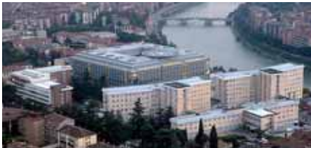
Trento Civil Hospital - Trento, Italy
